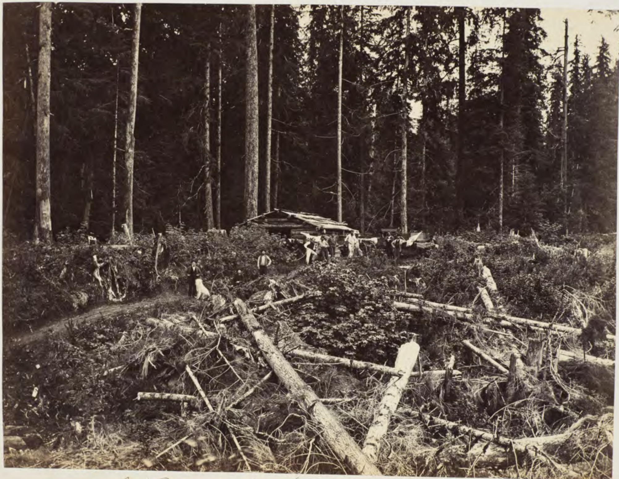
A View of the Woods at Merras's Inlet - B.C. 9014
