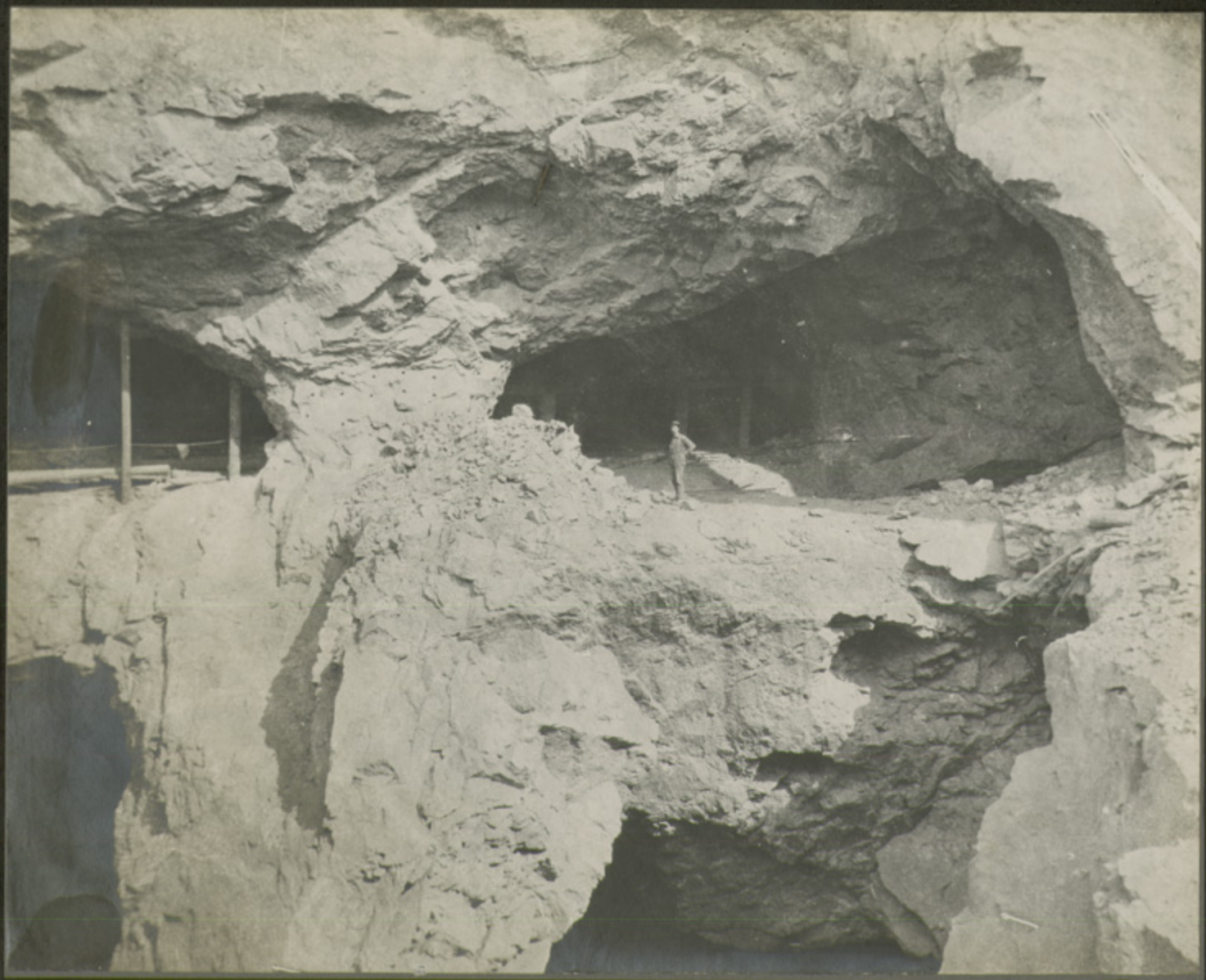
No. 2 Tunnel Stopes 1905.
