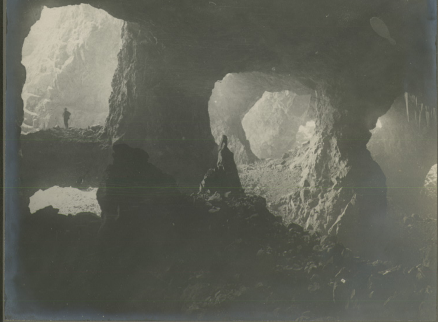
No. 2 Tunnel Stopes 1900 -
