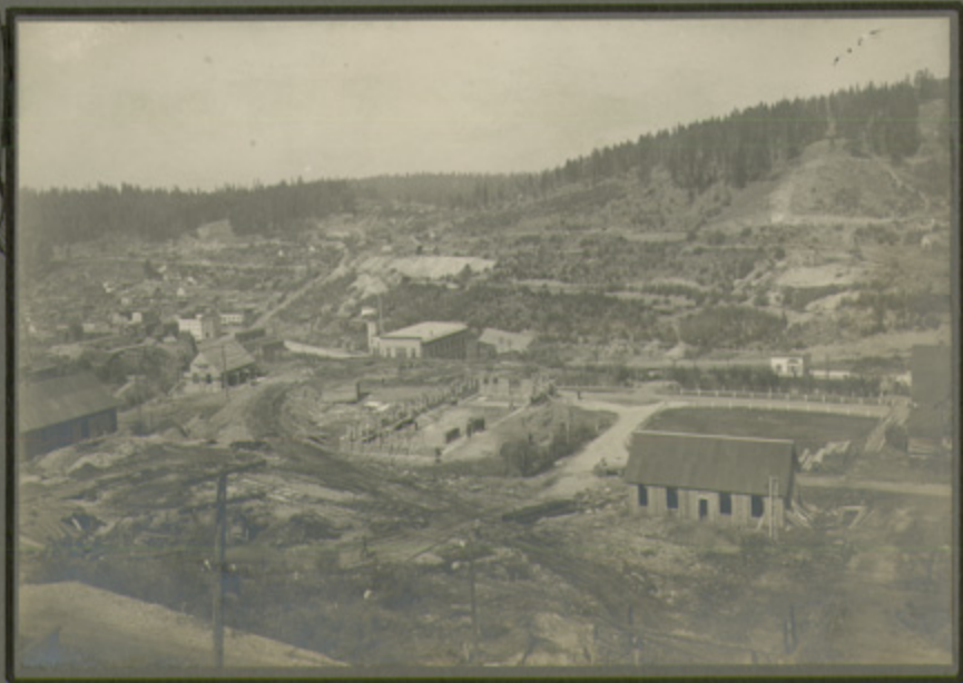
After the fire of Aug. 12, 1910-
