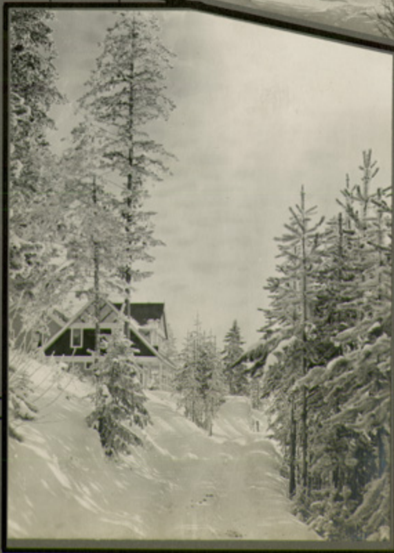
Snowshoe Cottage -- Superintendent's Residence
