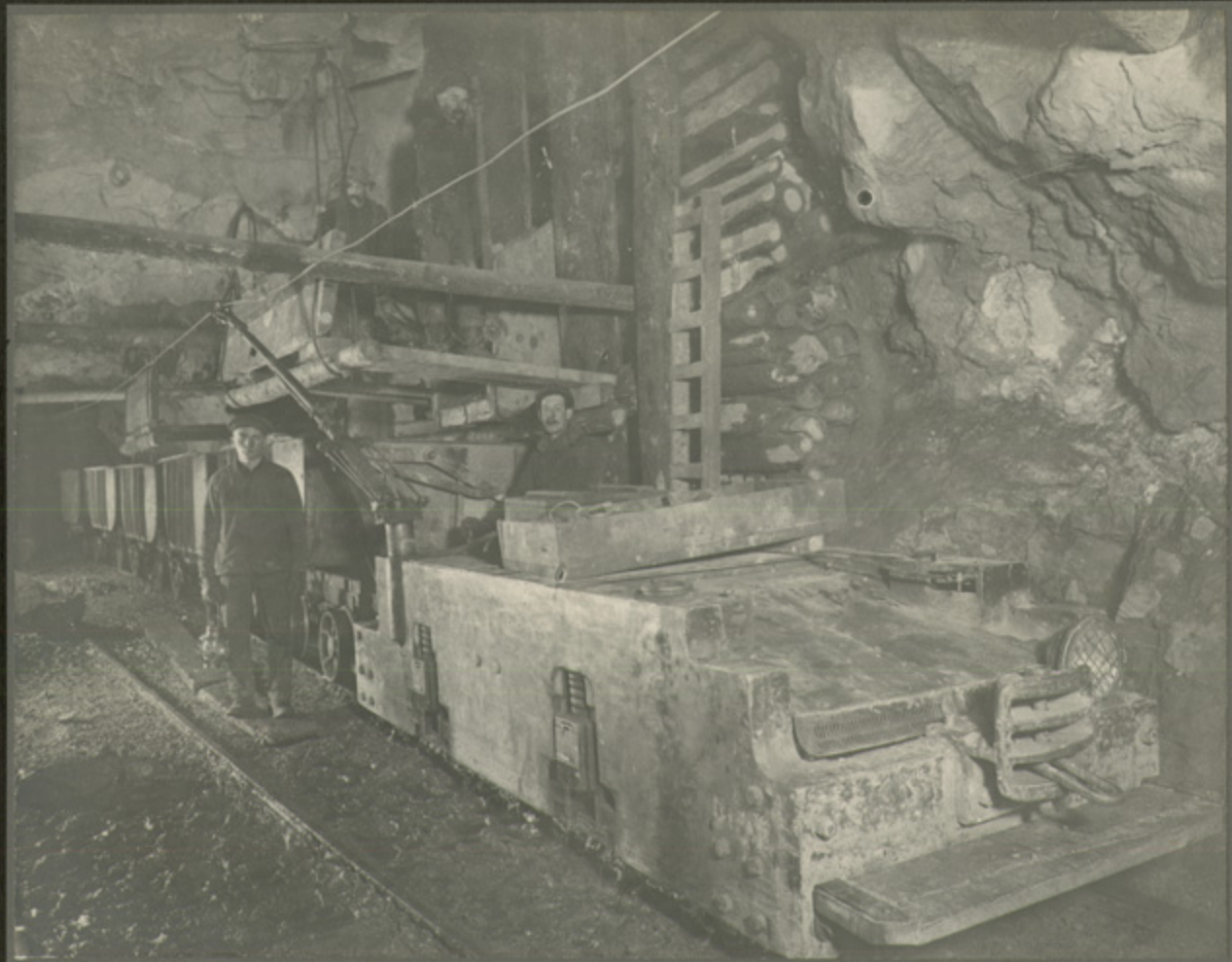
Loading Ore from Chutes 400' Level—
