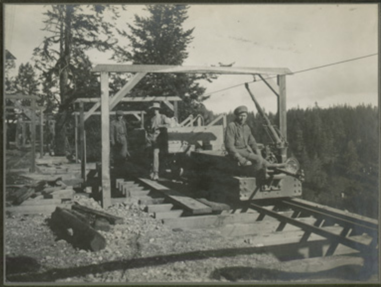
Mine Train No. 3 Tunnel—
