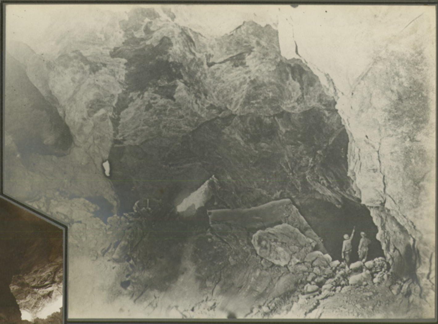
GOLD DROP MAIN STOPE Made by Removing Pillars at Right in No. 1. There are the same at Centre and Left in No. 2. Average Length, 400'; Width, 150'; Height, 80'; Ore Extracted, 400,000 tons.
