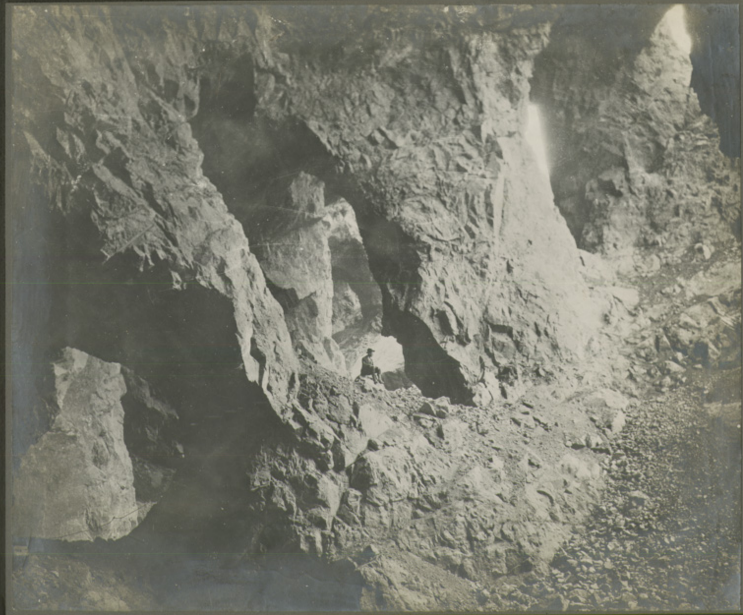
No. 2 Tunnel Slopes 1900
